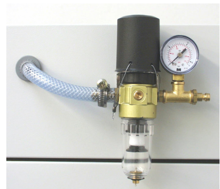
Figure 13: Compressed air connection with condensate separator
